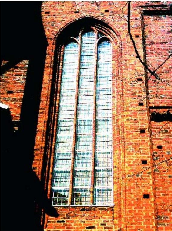
Figure 4: Protective glazing in Stendal, Germany<sup>8</sup>.
