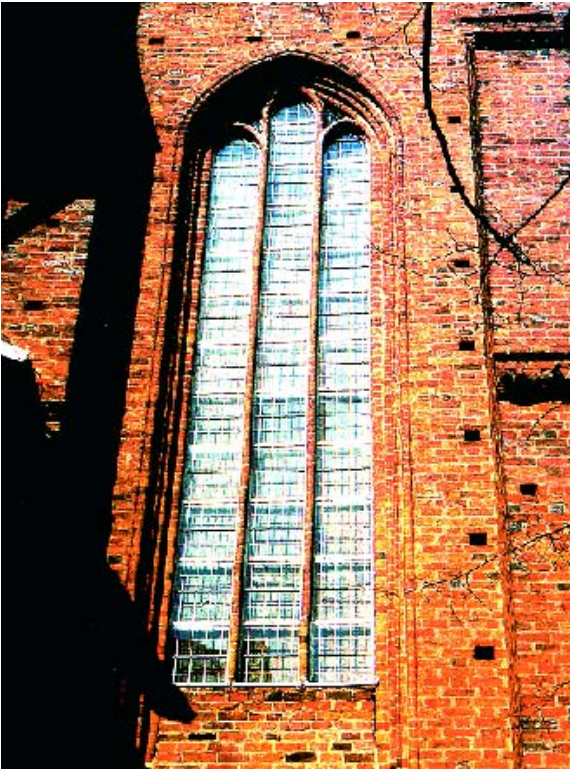
Figure 4: Protective glazing in Stendal, Germany 8 .
