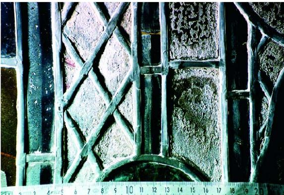
Figure 2: Detail of a stained glass panel from the Dome in Altenberg, Germany; the density of the corrosion crust depends on the composition of the glass and thus varies within one panel (photograph provided by the Dombauhütte Köln, Germany)
