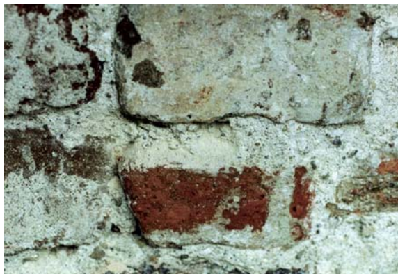
Figure 1: Left: layered plaster decayed by erosion, the upper layer is on the left, the inner layer (grey) on the right. Right: brick masonry with irregular mortar joints.
