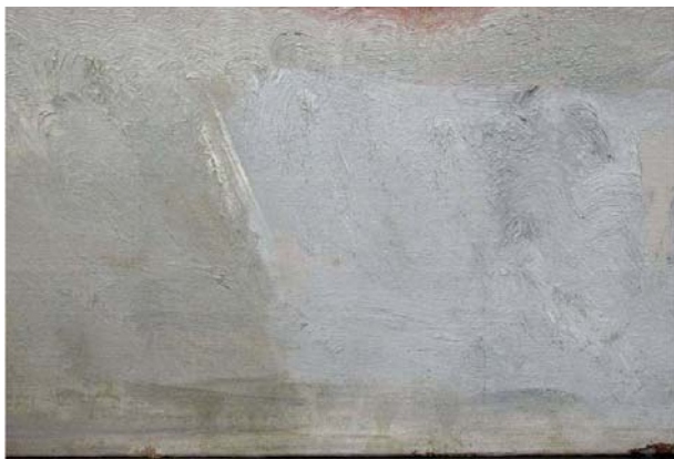
Figure 19: Detail showing area before and after cleaning with solvent gel.
