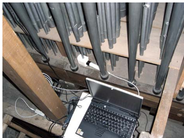
Figure 6b: System in operation in the Minor Basilica of St. Andrew the Apostle, Olkusz.
