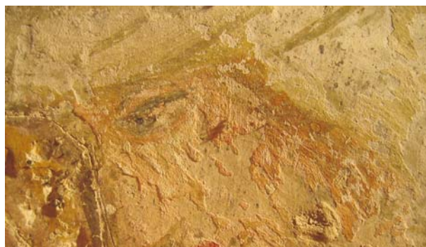
Figure 7: The thick layer of lime-wash falling from the wall together with overlaid paint layers, from Feistritz an der Drau.
